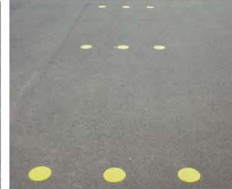
desactivated concrete, thermoplastic dots (crossings, parking signage)
